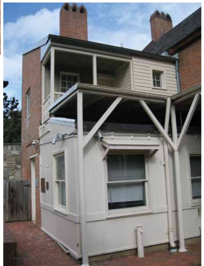
Top: the restored balcony. Right: before work began.
