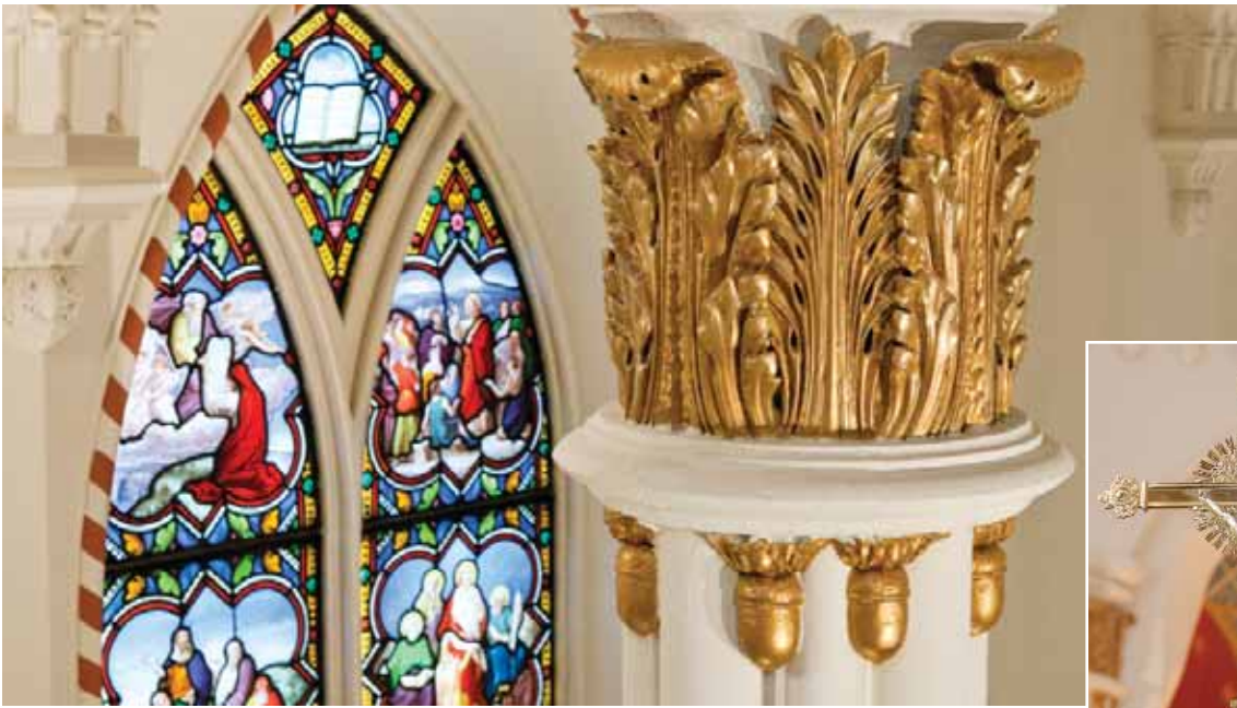
Restored columns and stained glass windows
